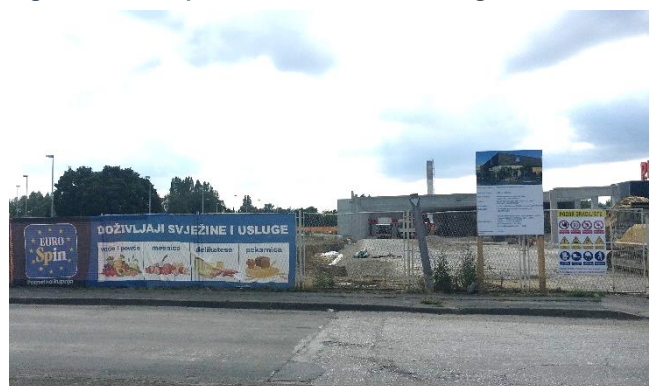
Figure 11: Eurospin construction site in Zagreb
